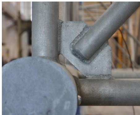
Figure 3.3: Intra-panel tertiary member detail; stiffener plate.
